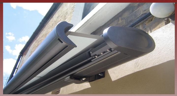
Designed with the idea of flexbility and durability in mind, this system will completely hide the fabric of the awning in a full casette, so that it won't get dirty or damaged while not in use. Modularity allows for diverse sensors to be attached to the system, so you will never have to worry about opening/closing it yourself.
